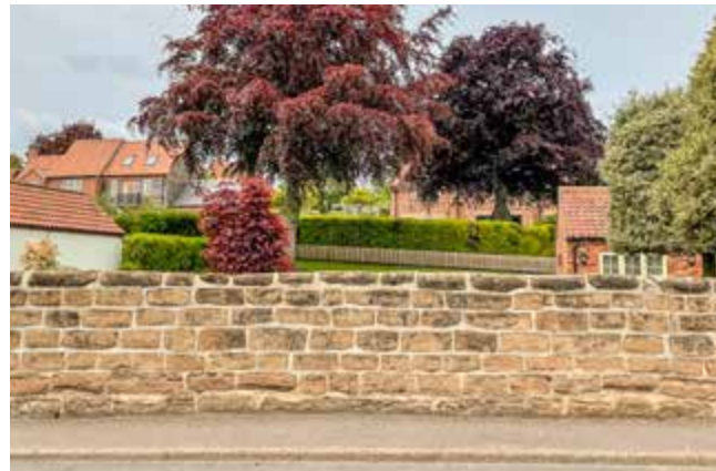
Stone boundary wall enclosing a garden in Woodborough contributes to street character
